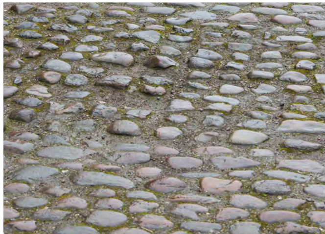
The type of pointing should be considered when identifying possible solutions for cobbled surfaces.
