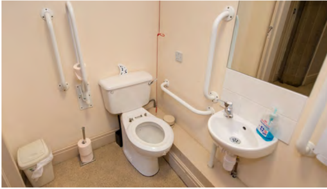
Choosing a suitable slip-resistant floor might be possible when making alterations in the historic built environment.
